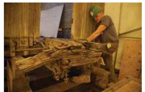
Wood was ordered and delivered for the new side sills, including two lap joints to make up the 37+ foot sill lengths.
