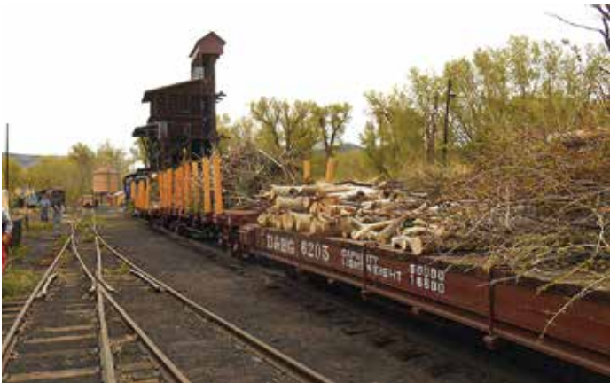
Returning to Chama, the work train backed down to the stock pens where the debris was unloaded for final disposal.
