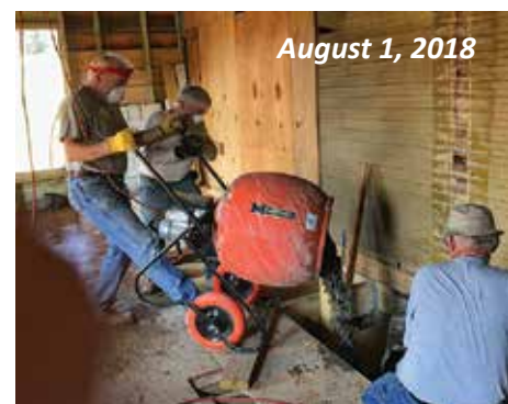
The original chimney foundation is gone and a new, reinforced foundation was poured in its place.
