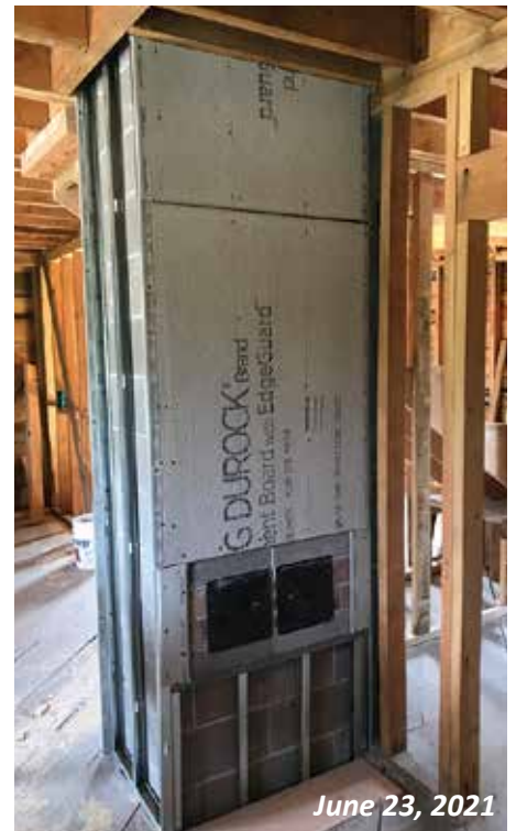
Inside, “backer board” was applied to the chimney for a plaster facade resembling the original facade.
