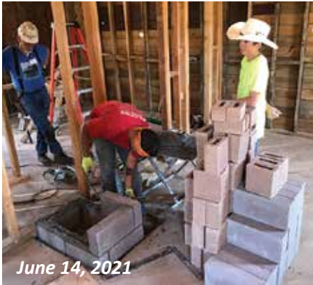
Wildfire Masonry arrived in June to begin construction of the new chimney, beginning on the first floor chimney pedestal.
