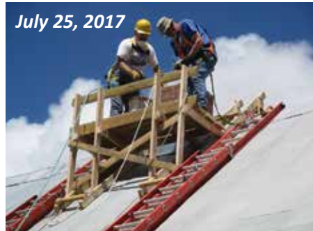
The roof of the Car Inspector's House has a 12:12 pitch, that is 45°. A platform was built to provide a safe work space.
