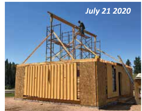
Like an Amish barnraising, the walls were lifted into place and their corners reinforced with OSB panels.
