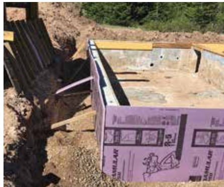
Rigid foam insulation protects the foundation from the frozen ground.
