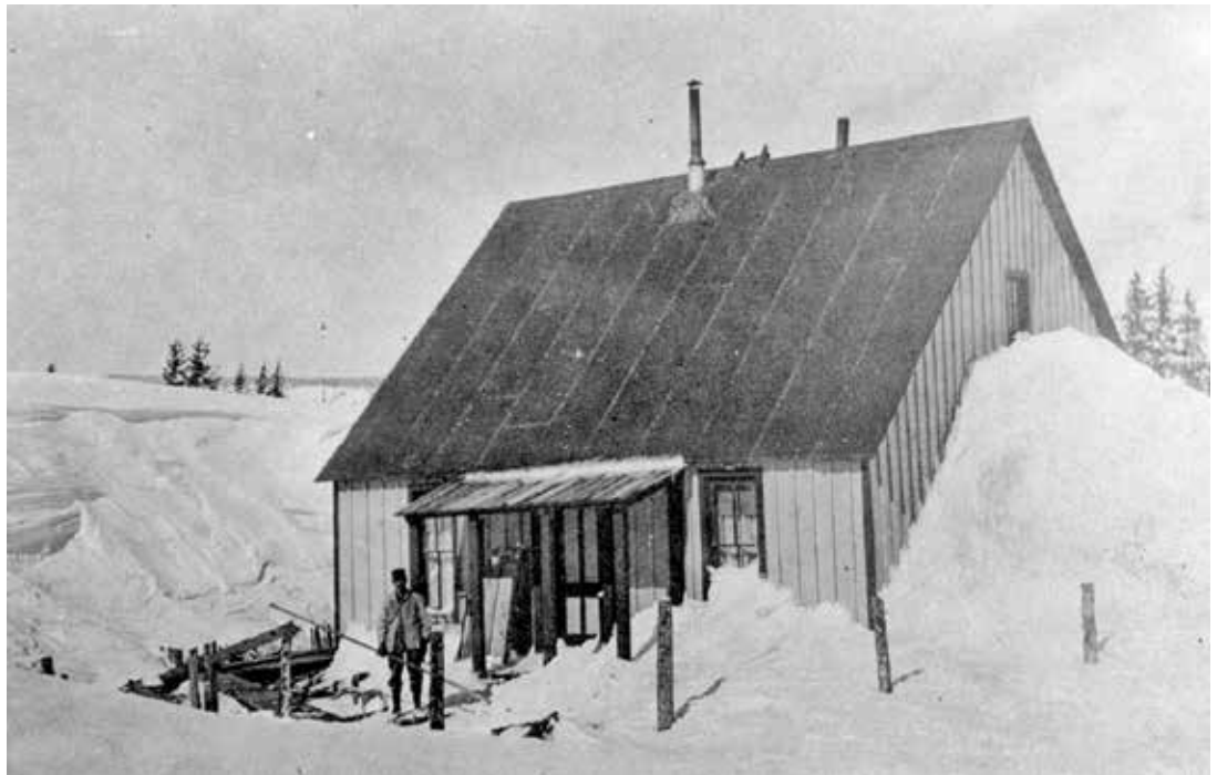
The Cumbres Car Inspector's House, ca. 1917, six years after its construction.
