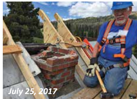
Like masons in reverse, John Pierce, Vance Behr and George Trever broke each brick free of the chimney's bonding mortar.
