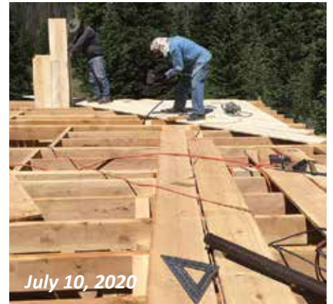
The concrete foundation, the first floor joists and decking, and the interior and exterior load-bearing walls will support not only the second floor but also the roof.
