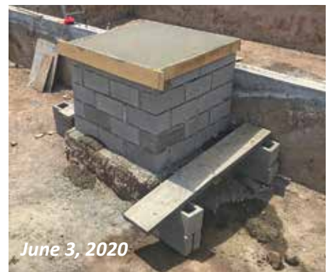
The pedestal will support the two-story, two-flue chimney.
