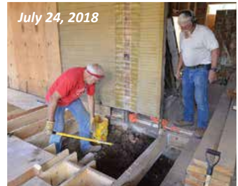
Like masons in reverse, John Pierce, Vance Behr and George Trever broke each brick free of the chimney's bonding mortar.
