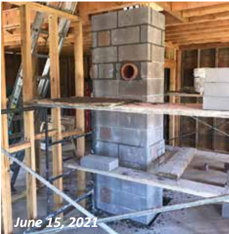
Wildfire Masonry arrived in June to begin construction of the new chimney, beginning on the first floor chimney pedestal.
