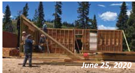
Like an Amish barnraising, the walls were lifted into place and their corners reinforced with OSB panels.
