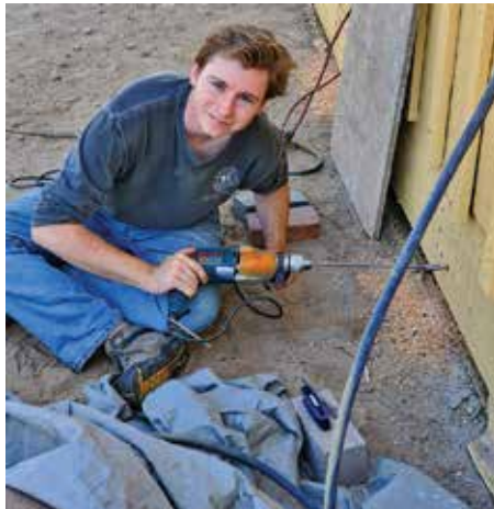
Remington Templeton part way through drilling 244 holes.
