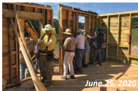
The concrete foundation, the first floor joists and decking, and the interior and exterior load-bearing walls will support not only the second floor but also the roof.
