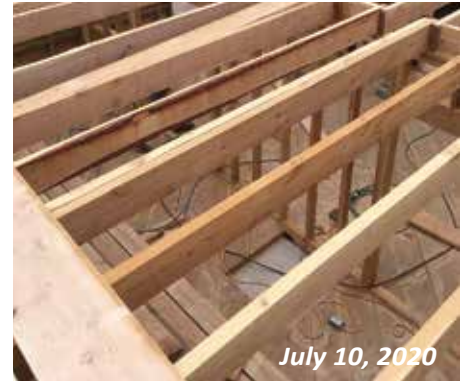
The concrete foundation, the first floor joists and decking, and the interior and exterior load-bearing walls will support not only the second floor but also the roof.
