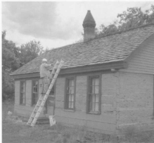
Bob Craine spraying on a heavy coat of Messmer's U.V. Plus "Natural" preservative.
