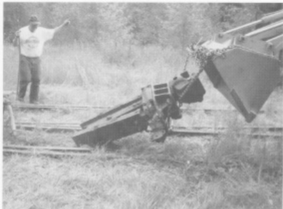
Don Bayer directs the removal of one of the stock car 5510 couplers. Both couplers were transported to Antonito.
