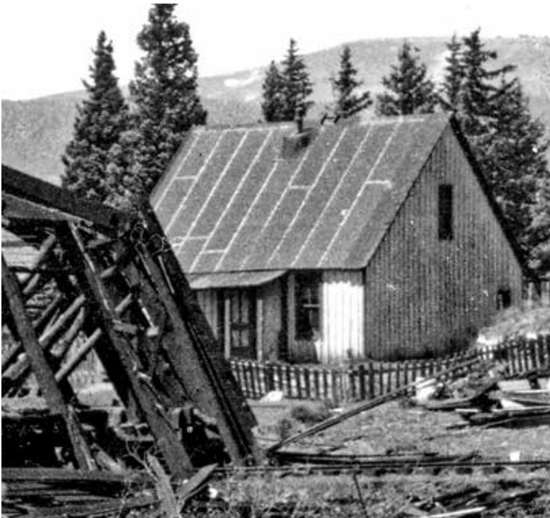
This is a portion of a photo taken to show the 1922 dismantling of the snowshed that covered the turntable. The Car Inspector's House looks fairly civilized, especially with the addition of a picket fence.
