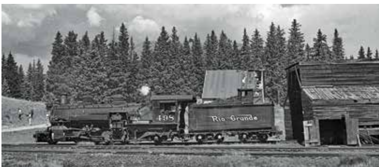
Forty-three years later, in 1965, the structure was showing its age. Portions of the roof have deteriorated down to bare boards.
