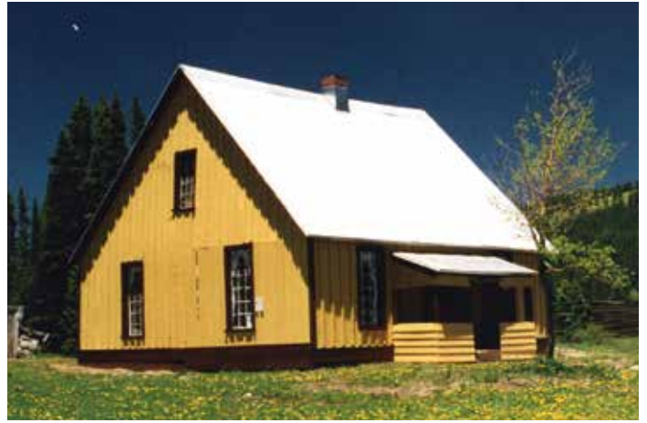
Not ready for occupancy, but by the end of the summer of 1995 the Car inspector's House was a much nicer looking piece of real estate and much more likely to remain standing. Photo by Glenn Hall
