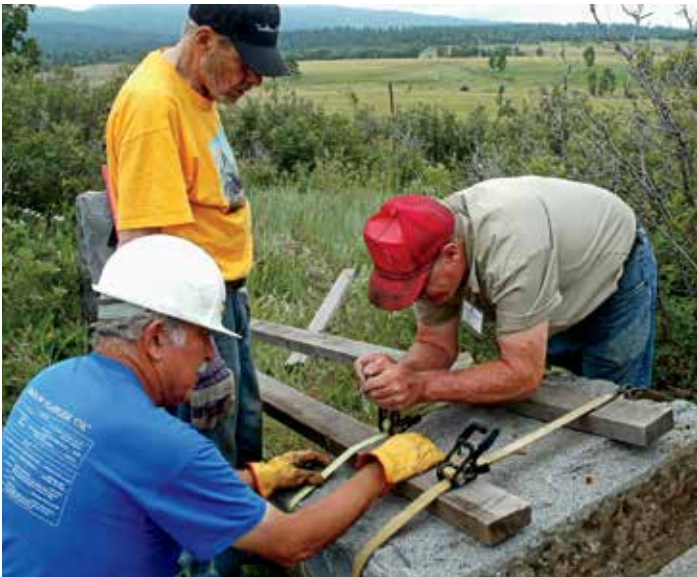
Bob straps eight-foot 2 x 4s to the tombstone with ratchet clamps. They will need all the leverage they can muster to tip the heavy headstone back into place.
