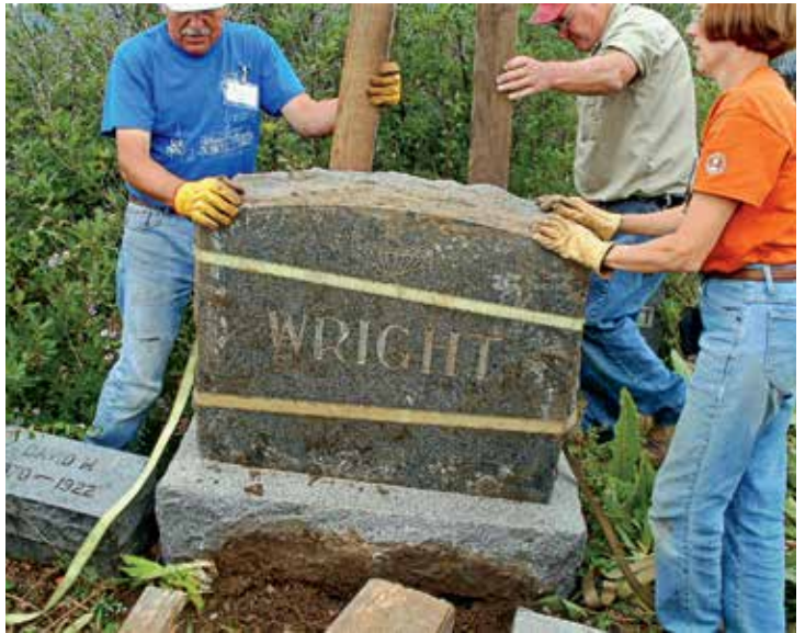
The tombstone is lifted back on to its base and is centered and stabilized.
