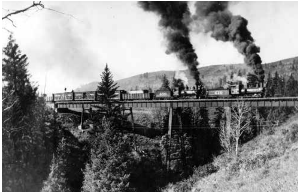
Locomotives 419 and 406 pull a stock train across Lobato Trestle, ca. 1908. Later No. 406 was renumbered 346 and is preserved at the Colorado Railroad Museum.
