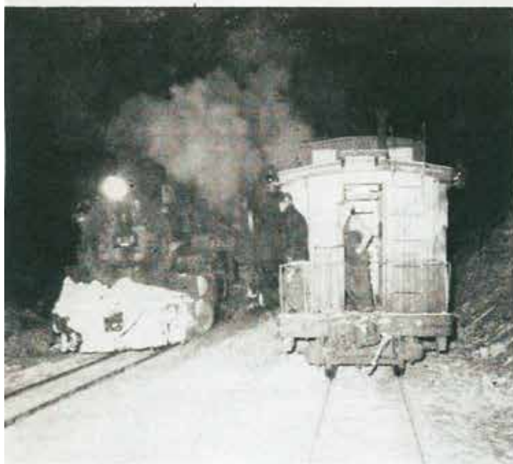
MEET with Extra 494 East . . . "no sight of glowing brake shoes — just the quiet clackety-clack of the joints."
