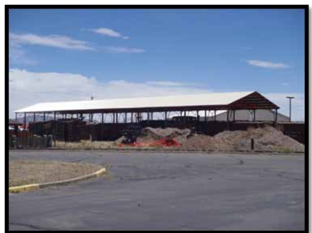
All of the roof panels are now installed!
