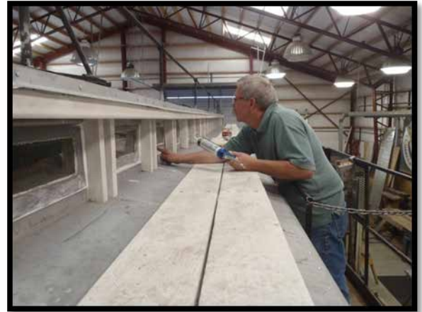
Mick O’Nele caulks around the clerestory windows
