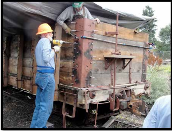
Warren Ringer drills another hole as John Sutkus tightens another bolt
