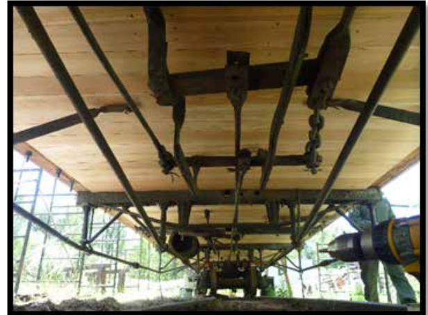
The undercarriage of the RPO 54. It hurts one’s back just looking at the work that was done upside down!
