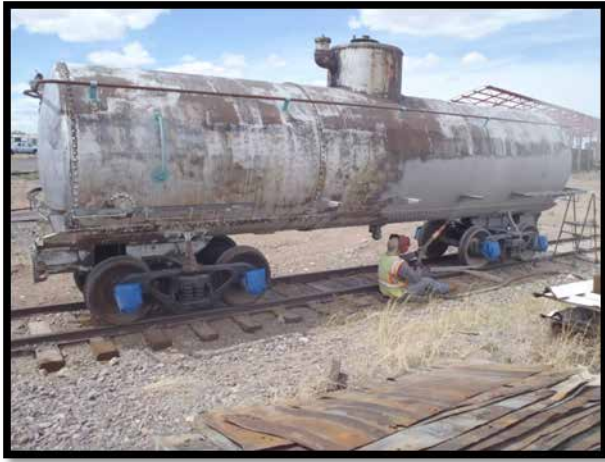
An outside contractor sand blasts one of the two Gramps frameless tank cars
