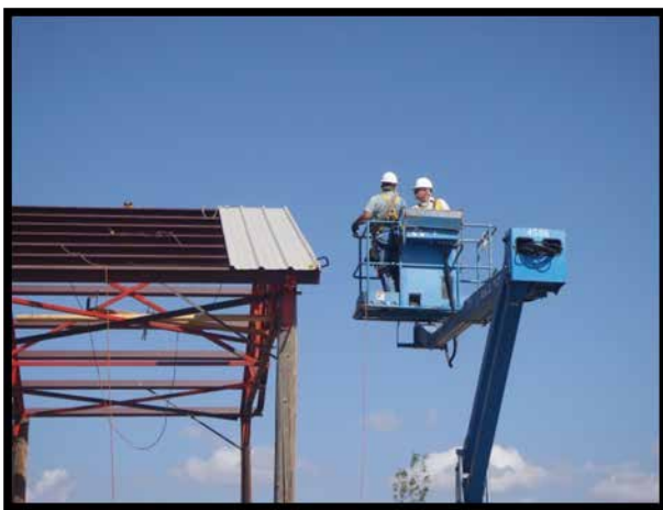
The first roof panel is clamped in place
