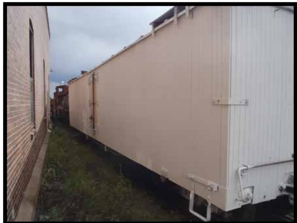
New siding had been installed and primed
