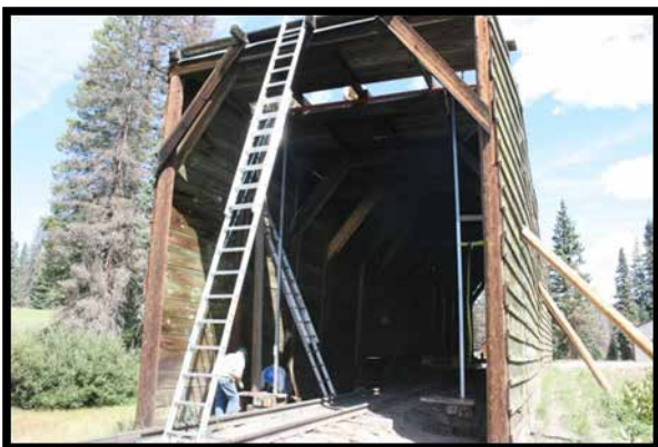
Metal temporary supports were installed
