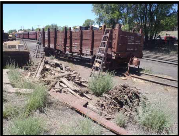
The two piles of trash wood show the condition of the floor and a few side boards
