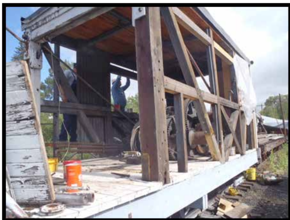
Old siding has been removed from the cabin
