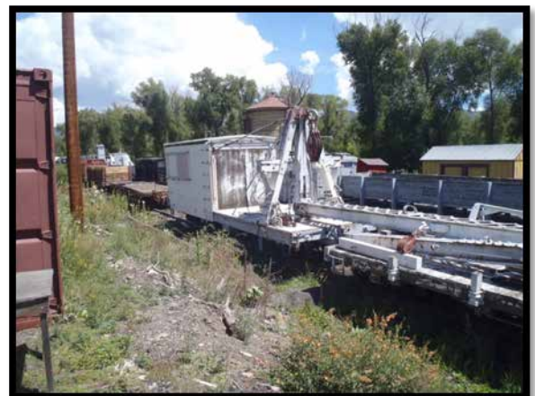
OP cabin with new siding and primed.
