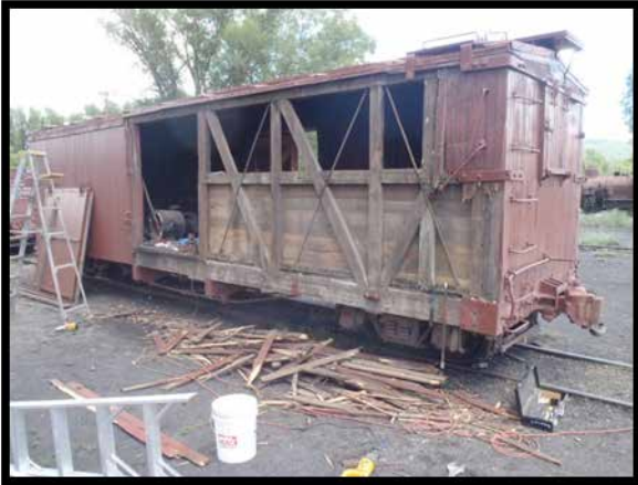
Most of the siding has been removed
