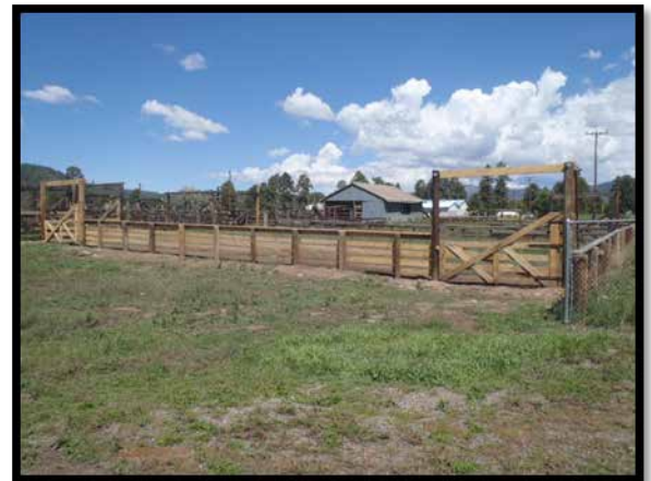
By Session F, the fence and two large gates were installed
