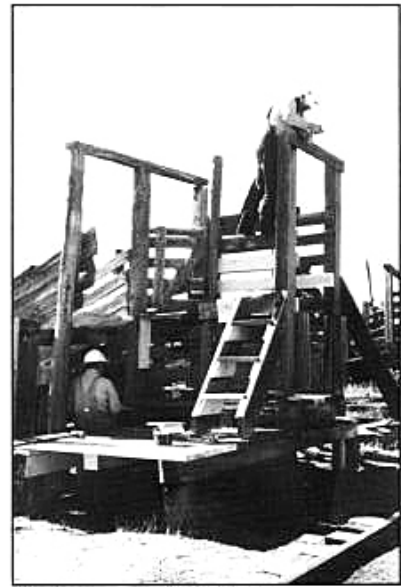
Repairs were made to the landings, ladders, and loading chutes of the stock pens at the south end of the Chama yard. August 1993. Photograph by Jessica Ratliff.
