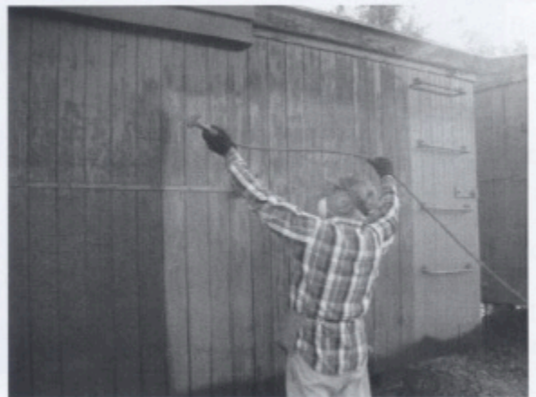
Bob Rosenberger applying the finish coat on boxcar 4342.
