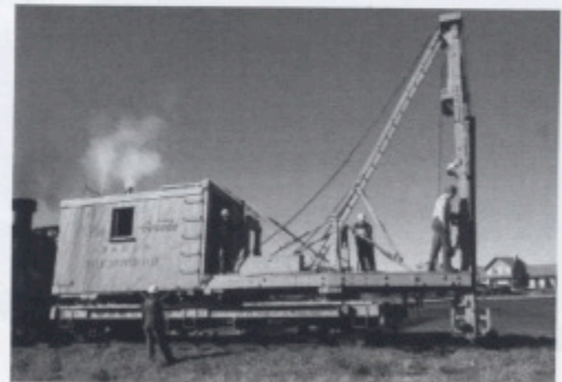
Pile Driver OB in operation as part of the TRAIN convention in October 2010.
