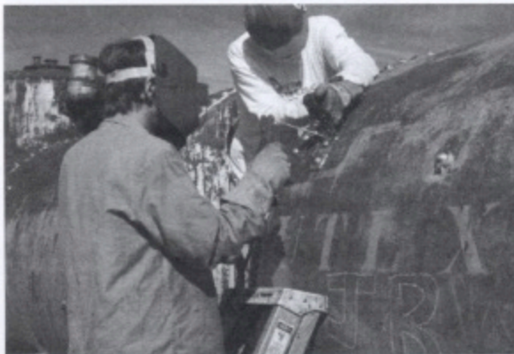
TL Chris Trunk tack welds first bracket while Kevin Pyle positions it.
