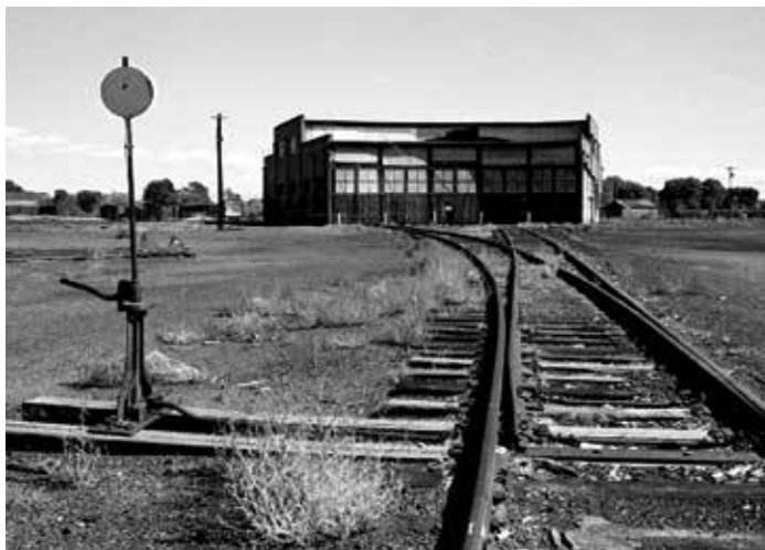
1994: The last remnant of the D&RGW's once-extensive engine facilities is the standard gauge section of the roundhouse. The shops and the narrow gauge portion of the roundhouse have been leveled. Even this fragment would soon be gone.
