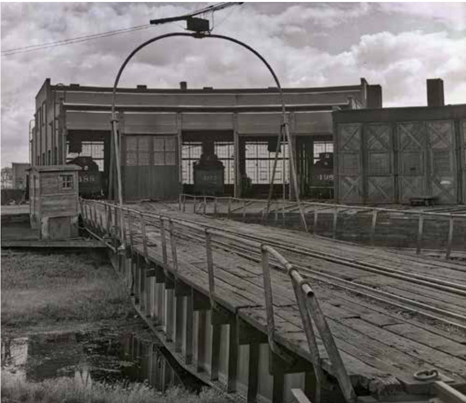
1964: The five bays of the standard-gauge section of the Alamosa roundhouse, bigger and better lit, have been modified to accommodate the almost-daily maintenance of the narrow-gauge locomotives, something the standard-gauge locomotives rarely need. Three have been converted to narrow-gauge, one remains standard and one is dual-gauge. The other stalls from the original slim-gauge days are still standing to the right of the brick structure during my 1964 visit.
