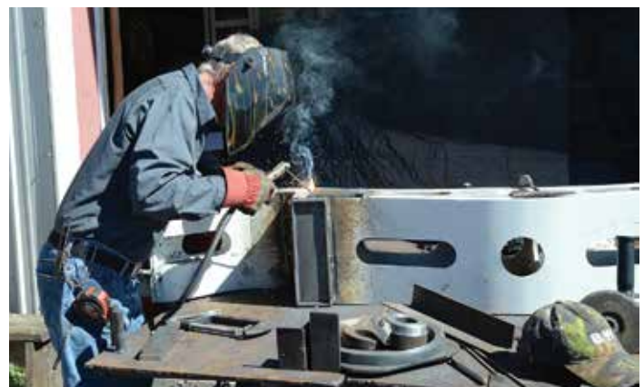
Welding on one of the two flying bolsters.
