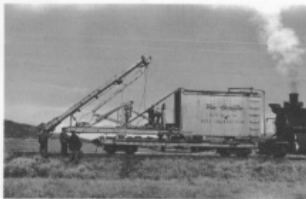
The boom of pile driver OB is lowered for movement between work sites. R.W. Richardson photograph. Date and location not certain. From the Richard L. Dorman Collection of Narrow Gauge Photographs.
