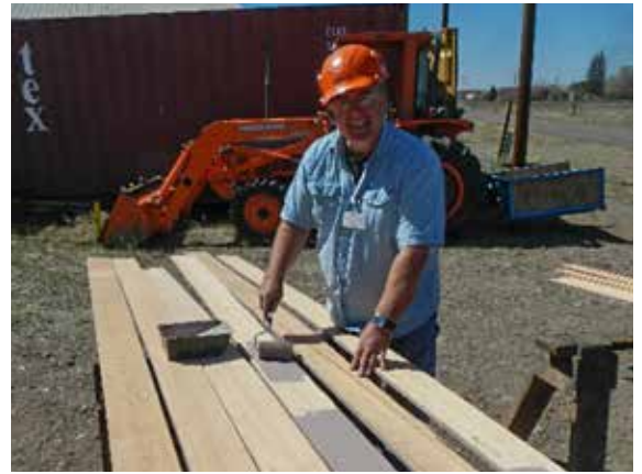
Bruce Bloom primes cedar siding for the Osier Section House.
