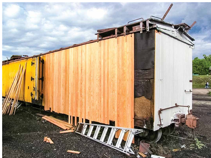
Partially repaneled Reefer 163
