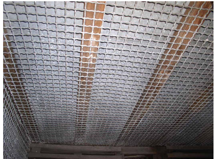
Caged steel lined wall of ice bunker
