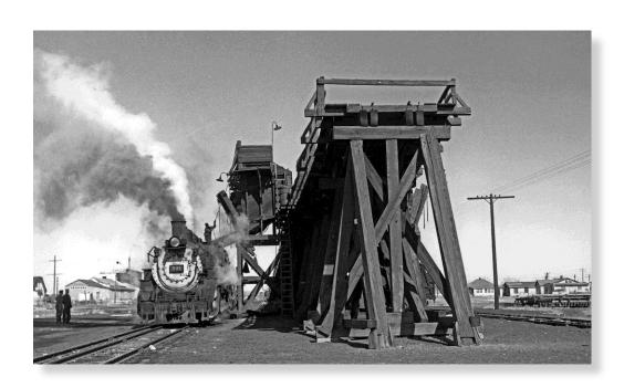
On February 20, 1956, Bob Richardson caught D&RGW K-36 #491's fireman attending to the loading of a tender-full of coal at the Antonito coaling trestle which was replaced by a "Red Devil" coal loader in the late 1950's. There were three elevated bins in this structure, presumably capable of refueling one engine each.
