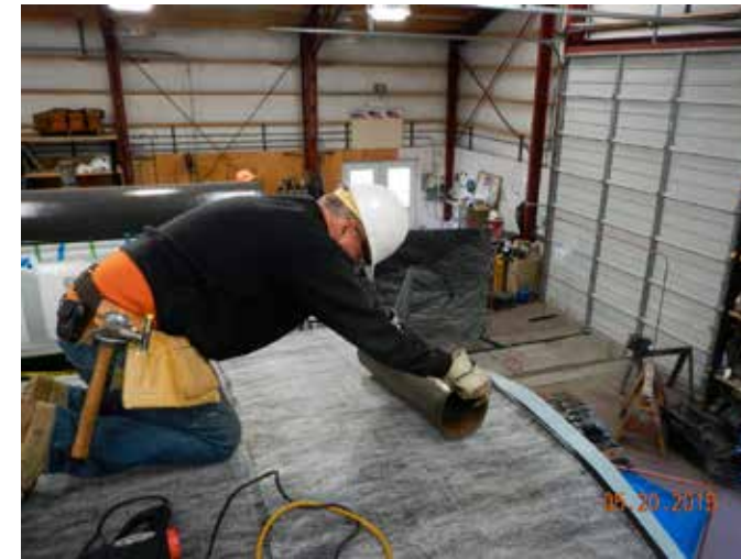
Double roof cover of snow and ice barrier.
