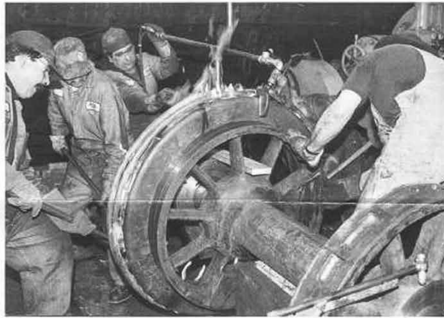
In the Chama enginehouse, the shop crew puts on a new tire for engine 463. The tire is heated with a "ring of fire" so it will expand enough to fit on the driver, with only a little coaxing from 15-lb sledge hammers. Left to right: Steve Montano, Toby Vigil, Orlando Uliberri, and Bob Wright. (March 2001.)
