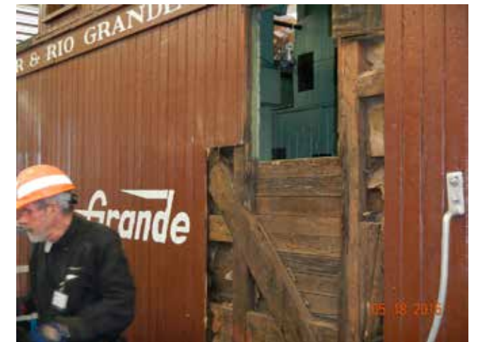
0579 Window water damage repair
